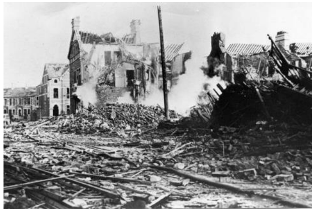
Figure 13 – Air raid damage to Neville St, Grangetown.
